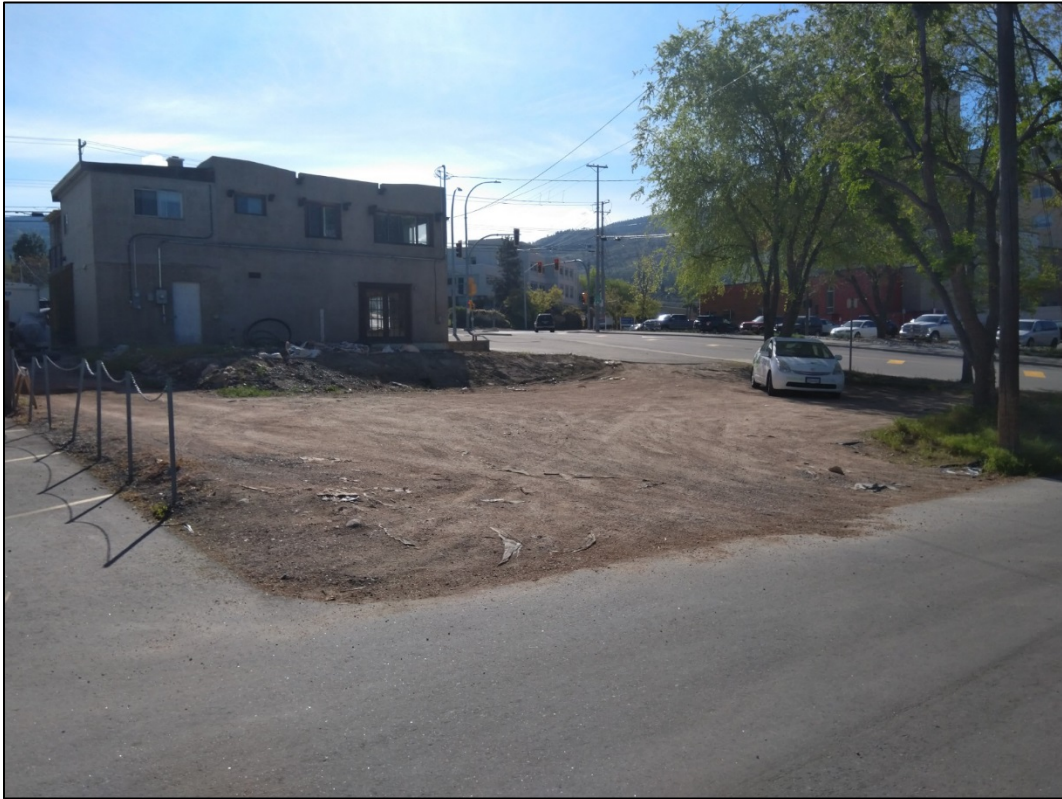
Figure 8: West view (from the lane)
